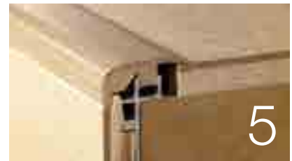
Stair nose moulding For a step down from a floating floor, e.g. at the top of the stairs or a step down in a room.
